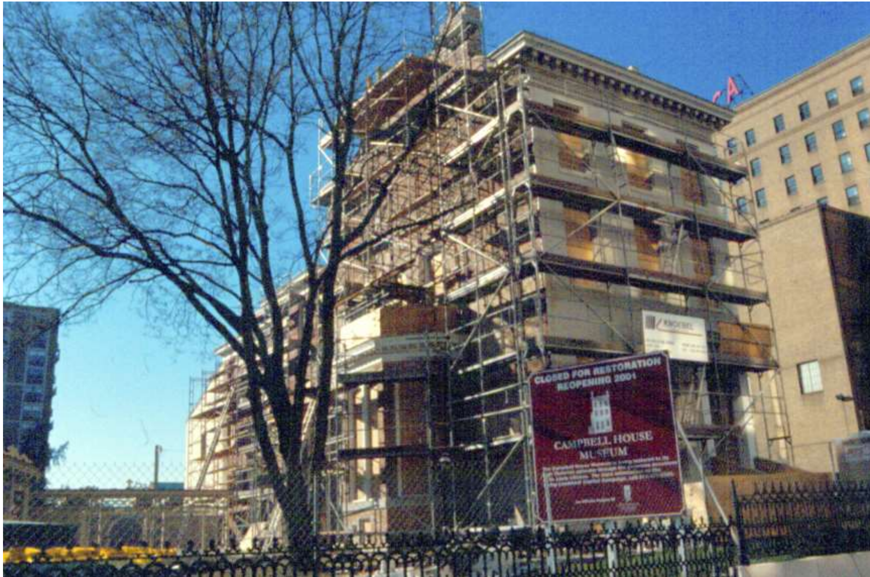
Front and east facades of house during restoration, circa 2001.
